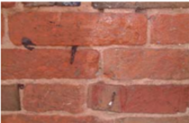
Photo illustrating an area of brickwork treated with Waterstop
