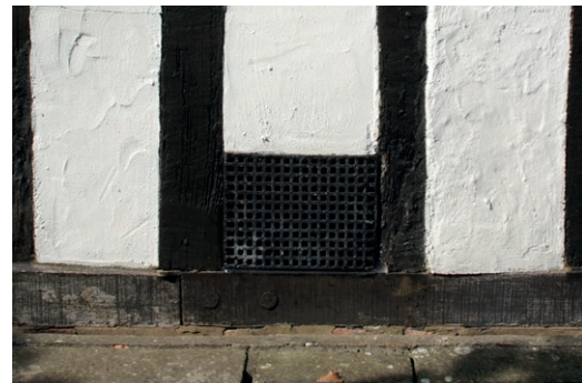
Flood Angel Double Anti-Flood Airbrick in black, installed behind the existing grill on this Grade II listed property.
