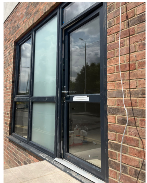
Photo showing BSI Kitemark™ Certified Flood Door with Low Threshold
