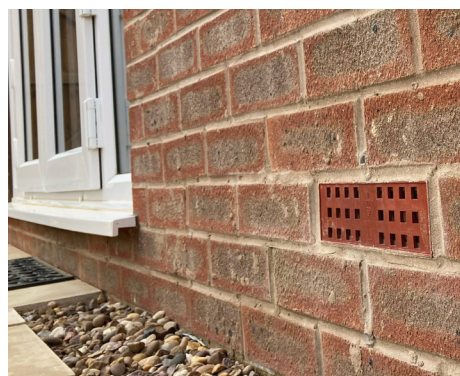
Flood French Door shown alongside installed antifoam airbrick
