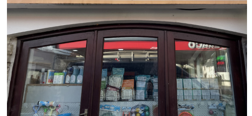
Photo showing arch detail on one of the large openings
