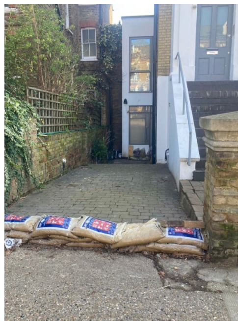
Photo showing homemade flood barrier used prior to installation
