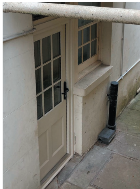
Photo showing Glazed Timber Door and Window below ground level
