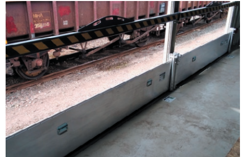
Photo showing barriers installed on carriage
