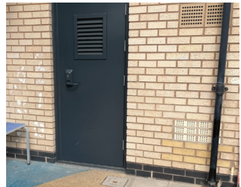
Photo shows Anti-flood Airbricks & Flood Defender Steel Door to plant room
