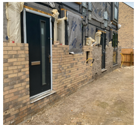
Photo showing Anti-flood Airbricks
