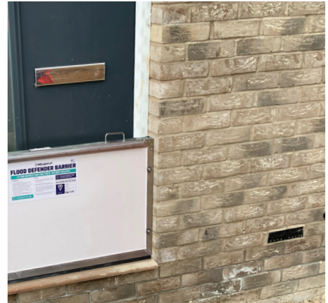
Photo showing Anti-flood Airbrick & Flood Defender Barrier
