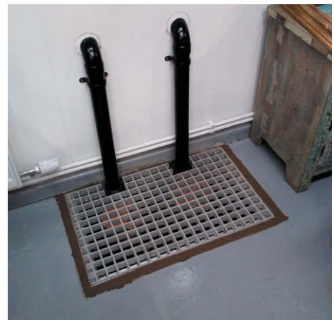
Sump & pump buried internally with mesh grill.
