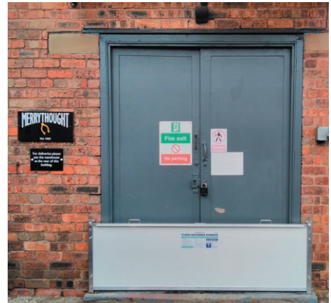
Flood Defender Barrier providing protection to fire exit.
