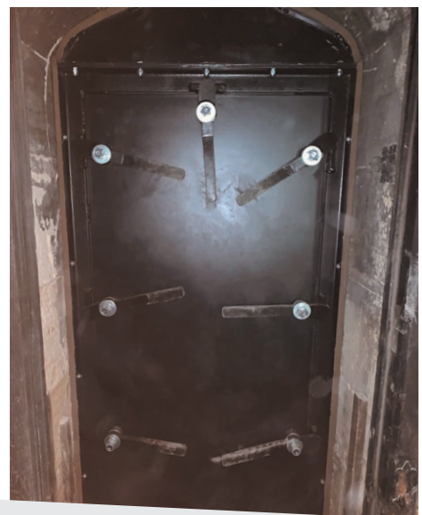
Existing 18th Century flood door replaced with 21st Century flood door
