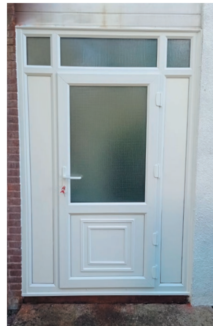
Photo showing rear white UPVC door and side panels
