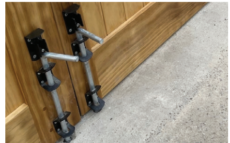
Photo showing drop bolts on inside of gates
