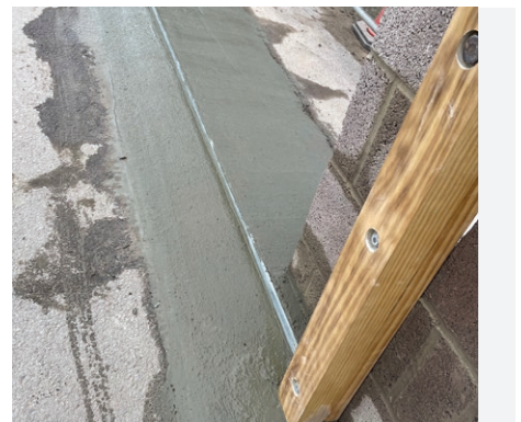
Photo showing groundworks and post during installation
