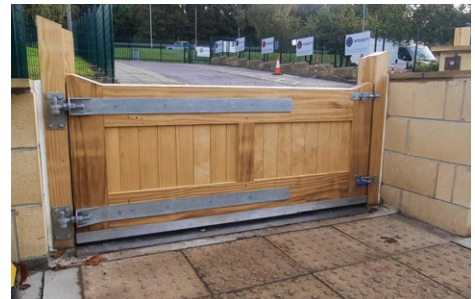
Photo showing DDA compliant threshold seal
