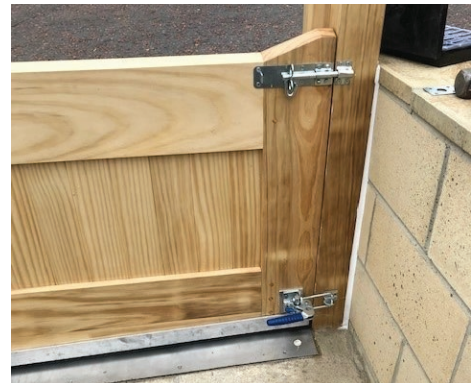
Photo showing toggle latch for extra security & seal closure
