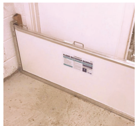
Defender Barrier installed in lower level entrance
