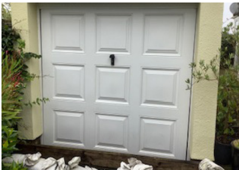
Photo shows garage door before Flood French Door Installation
