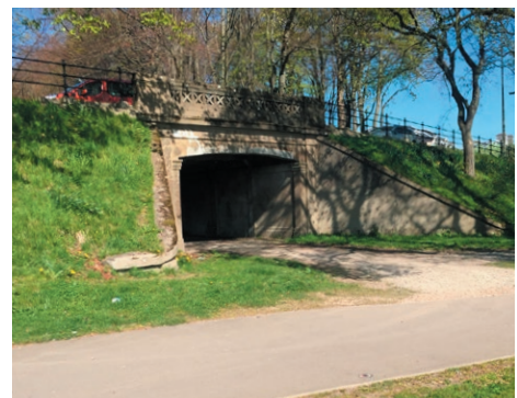
Underpass before OMO Flood & Storm Gate installation
