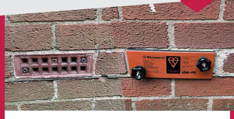
Located in East Yorkshire this property suffered years of damp beneath the floorboards as heavy rainfall build up seeped into the floor void through open airbricks.
