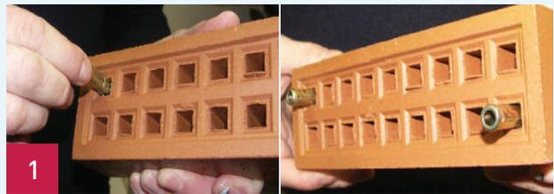
2. With a hammer gently tap the anchor bolt into the brick, as far as possible.
